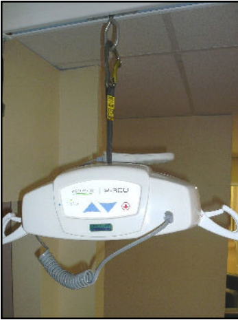
Figure 9A - Photo showing connection of lift hook directly to the eyelet of the trolley.
