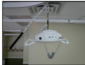
Figure 10A - Photo showing P-440 lift carabiner connected to a reacher first and then to the eyelet of the trolley.
