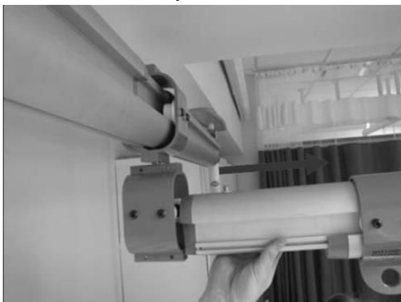
Figure 31: Remove the Traverse Track from the Trolley
